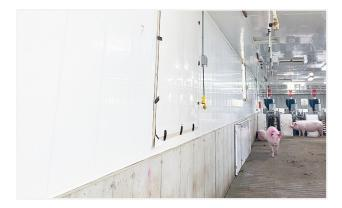
Use lightweight, non-porous Trusscore Wall&CeilingBoard for all load bearing walls and ceilings. It's easy to clean, can handle repeated pressure washing and withstand harsh gases in the air.
